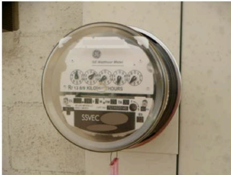
Analog meter with hidden PLC transmitter. The serial number has been blanked out to protect privacy.
